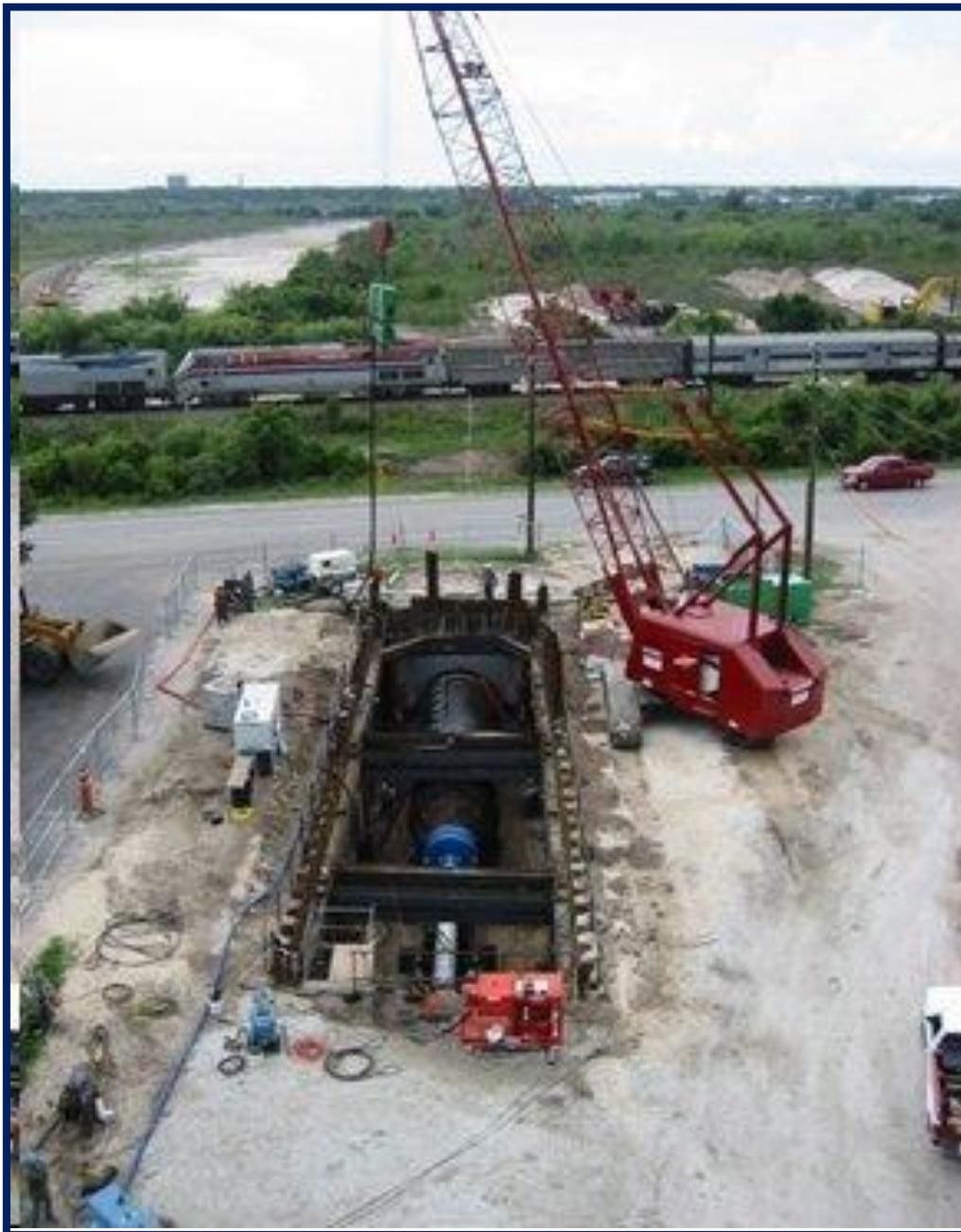
**Hydraulic Hammer for horizontal driving of a 3m diameter, 100m long pipe as a tunnel under a road and railroad track in Tampa - FL-EUA.**
