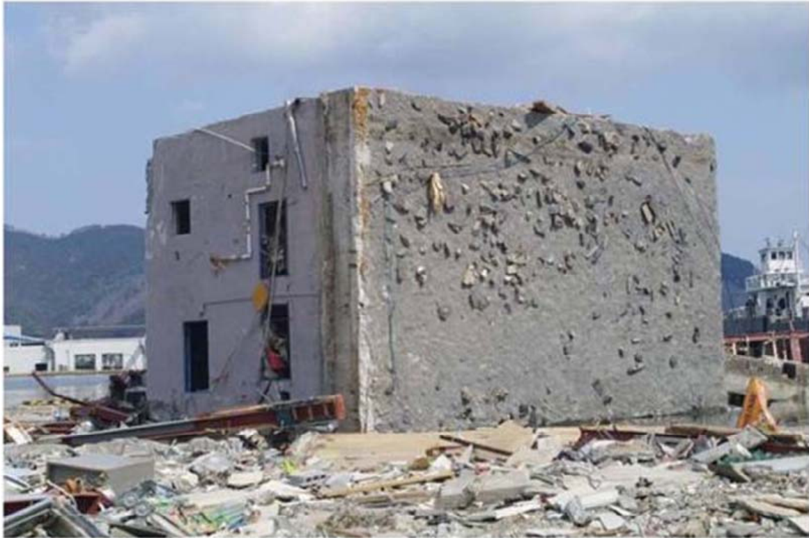
Overtured RC-building with shallow foundation. (Motoki Kazama, Tohoku University from Japanese Geotechnical Society (JGS) website : first results of its activities after the occurrence of the 11th March, 2011 Tohoku earthquake, http://www.jiban.or.jp/e/disaster-survey-information-of-2011-tohoku-earthquake-2/ )
