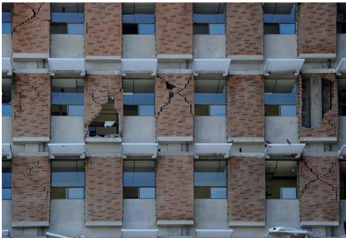
Fig. 10 Shear failure of non structural facade walls of the Monsenor Sanabria Hospital (Source: La Nacion, online version).
