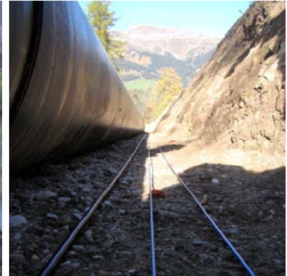
Figure 12: a) “Visible” landslide boundary: the leaning tower in the front is built on the moving area, while the tower in the back is on stable ground; b) Large, soil-embedded FO strain sensing project in the Swiss Alps for hydropower.
