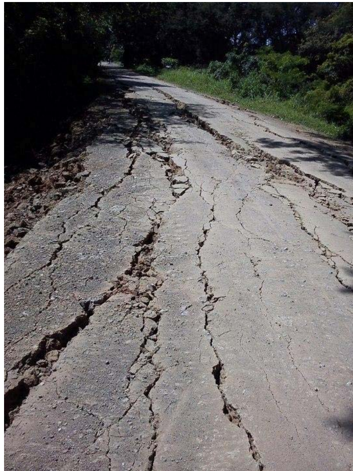
Fig. 8 Tension cracking and slope failure of the Tempisque levee at Filadelfia (Source: La Nacion, online version).
