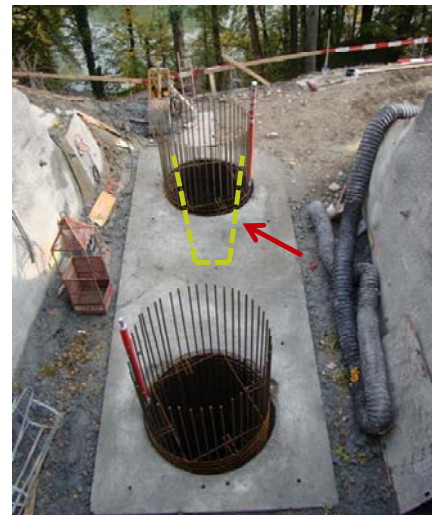
Figure 4: Two examples of construction sites in Switzerland which are instrumented with distributed FO strain sensors.
