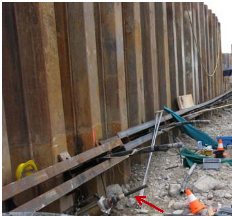
Figure 4: Two examples of construction sites in Switzerland which are instrumented with distributed FO strain sensors.
