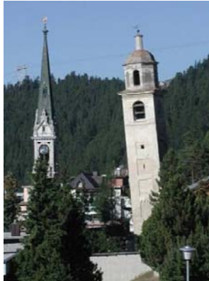
Figure 12: a) “Visible” landslide boundary: the leaning tower in the front is built on the moving area, while the tower in the back is on stable ground; b) Large, soil-embedded FO strain sensing project in the Swiss Alps for hydropower.
