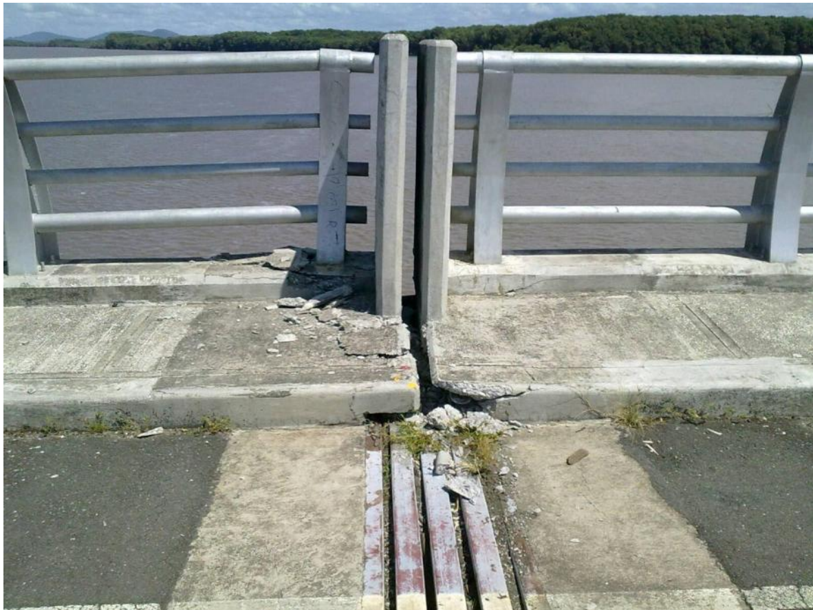
Fig. 9 Collision and permanent relative displacement between the two spans of the Amistad bridge (Source: La Nacion, online version).
