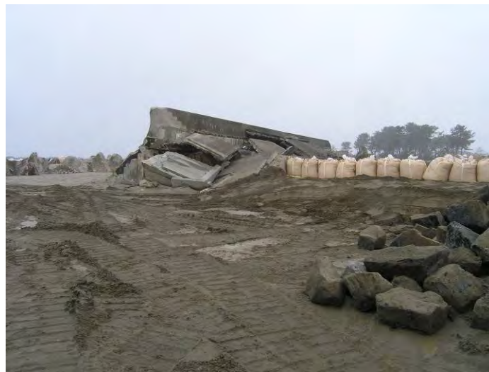
Fig. 13 Destroyed sea wall near Abukuma River mouth
