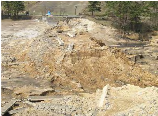
Fig. 41 Seismically breached Fujinuma Dam
