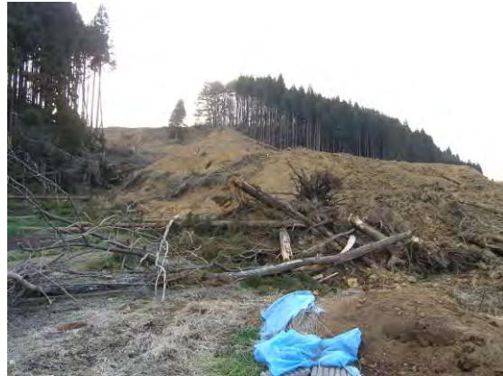
Fig. 32 Failure of natural slope at Hanokodaira of Shirakawa City
