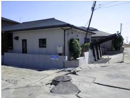
Fig. 29 Liquefaction-induced house damage in Hinode area of Itako City, Ibaraki
