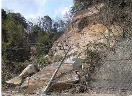
Fig. 31 Rock fall at Ohgo of Ibaraki
