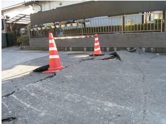
Fig. 16 Distortion of road pavement in residential area (Mihama of Chiba)
