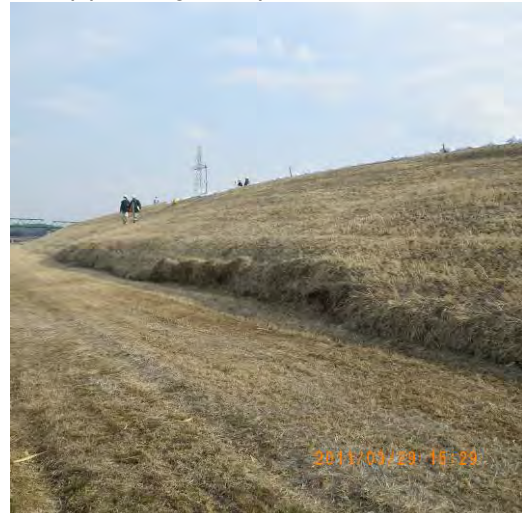
Fig. 26 Distortion of Naruse River levee on right bank near 40.0 km post
