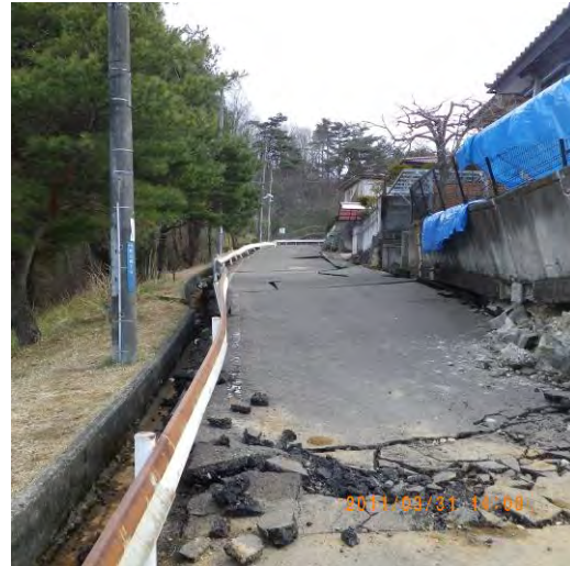
Fig. 39 Damage that was limited to filled part of residential development in hilly area (Oritate 4 of Sendai)
