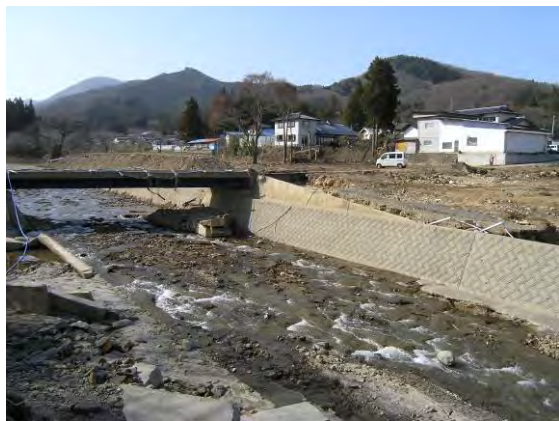
Fig. 43 Village attacked by flood
