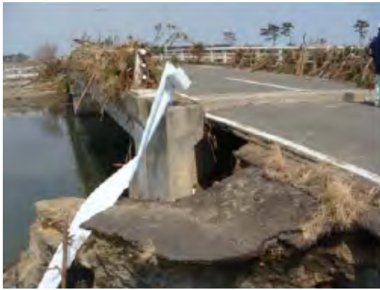
Fig. 11 Erosion of embankment at bridge abutment after tsunami Strike (Iwanuma in Miyagi Prefecture)
