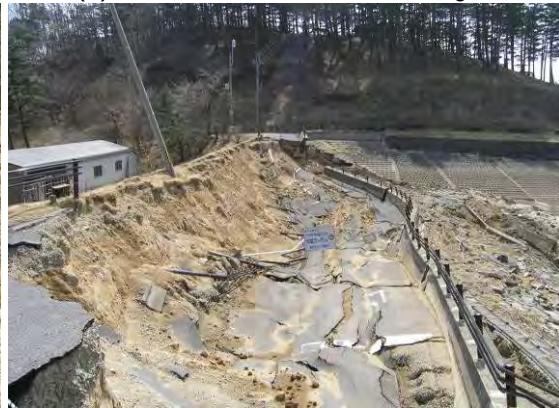
Fig. 41 Seismically breached Fujinuma Dam
