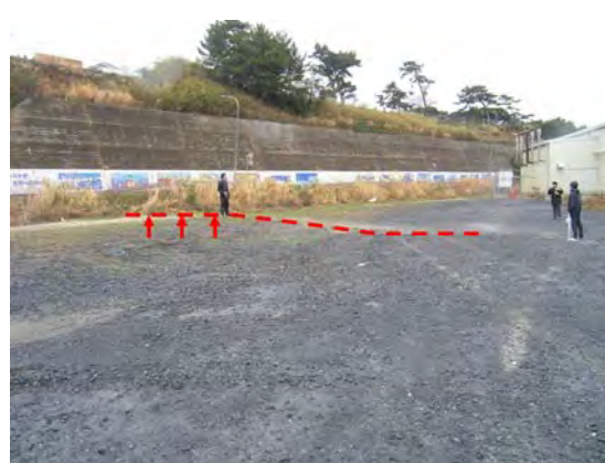
Fig. 22 Uplift near the toe of distorted slope in the previous figure
