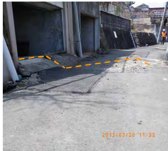
Fig. 37 Compressive distortion of ground surface near bottom of unstable slope (Midorigaoka of Sendai)
