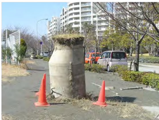
Fig. 18 Uplifting of manhole of 2 meter in Urayasu of Chiba
