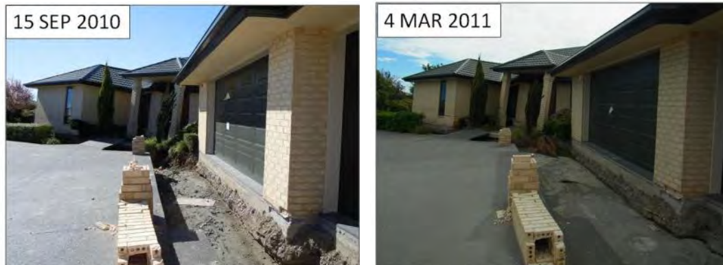
Figure 19. Minor additional damage to a residential house which underwent foundation failure due to lateral spreading and liquefaction in 2010 Darfield Earthquake. (South Kaiapoi)
