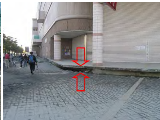
Fig. 15 45-cm subsidence of ground surface in front of a shopping center (Urayasu City)
