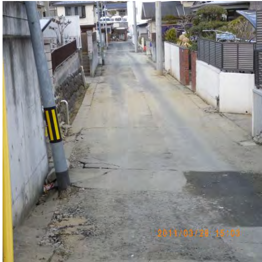
Fig. 38 Soil liquefaction in Asahigaoka 2 of Sendai City
