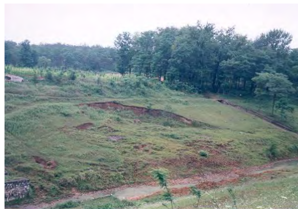
Figure 3 A typical failure of an expansive soil slope at Dagangpo
