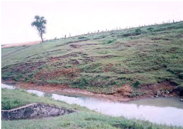
Figure 4 Typical shallow retrogressive failures at Dagangpo
