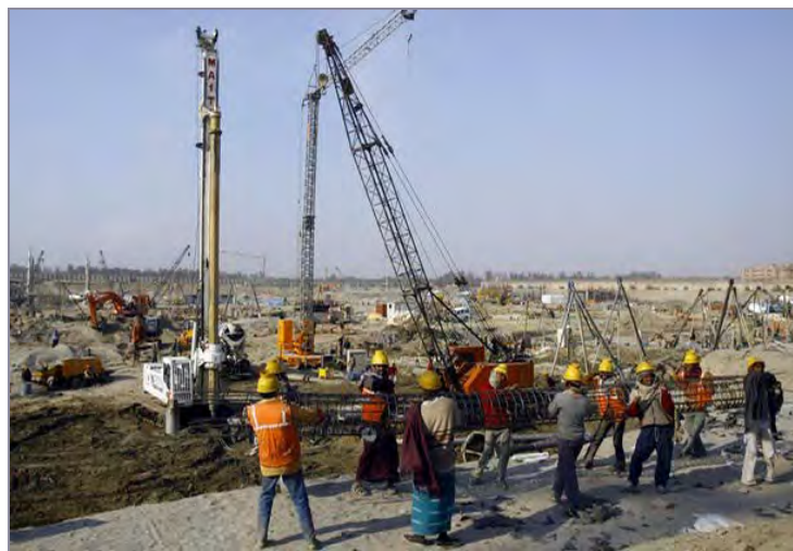
Figure 10 Piling in Progress at Site
