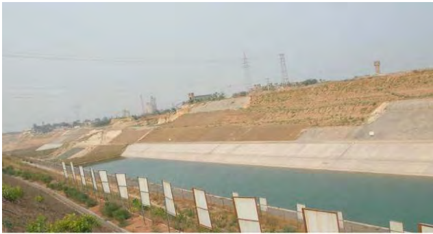
Figure 13 Part of Luwangfen test section in expansive soft rock (with courtesy of Professor Gong Bi-wei)
