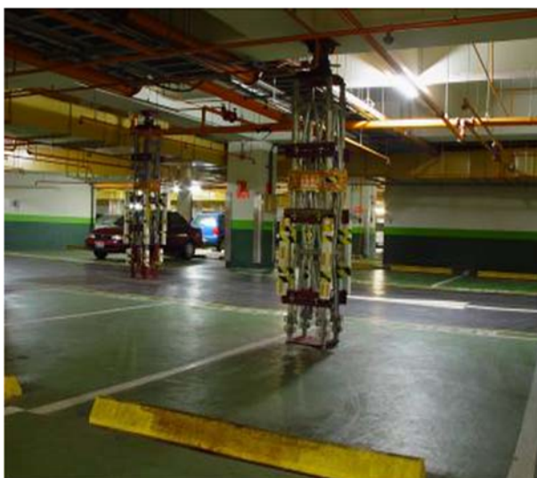
(a) Installation of underpinning of underground car park structure
