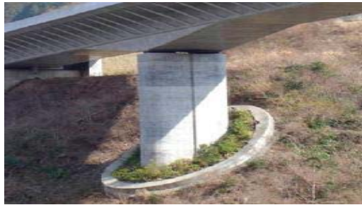
Figure 5 Photo of bamboo-cutting method of shaft foundation
