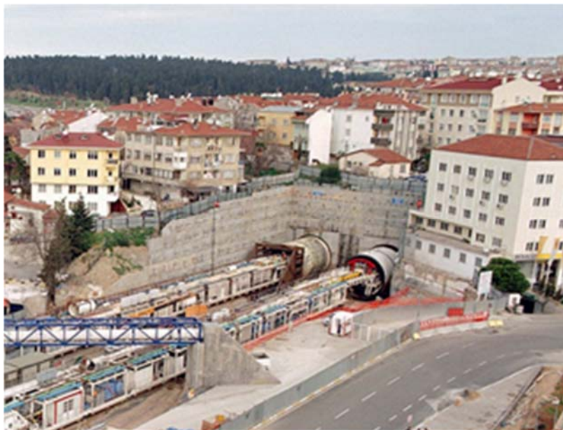
Fig. 5-2 Excavation in an urban area
